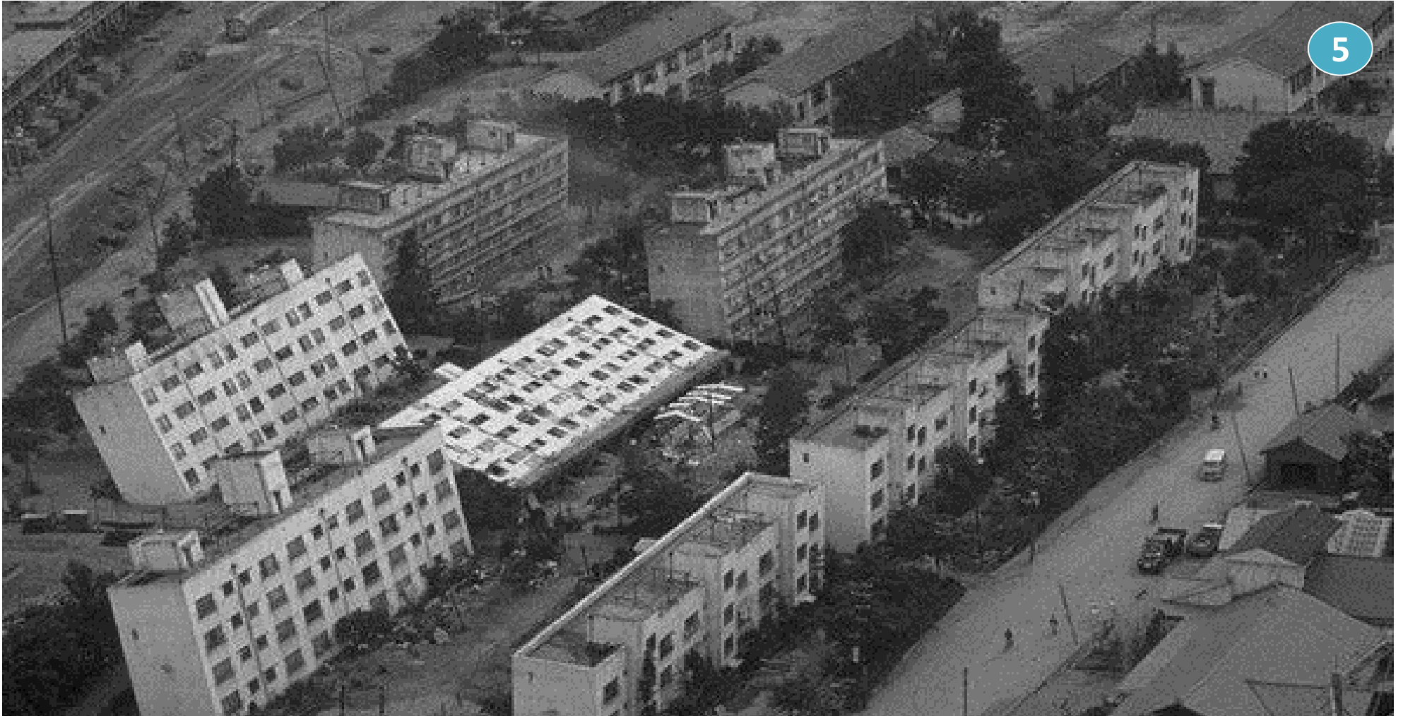
Fig. 7 Collapse of the apartment complex of Niigata prefecture. Source: https://goo.gl/zukWJh
