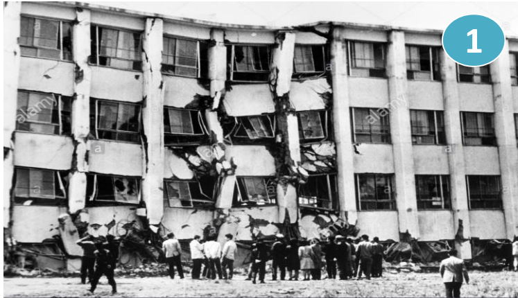
Fig. 3 Differential settlements Source: https://goo.gl/xYdCvb
