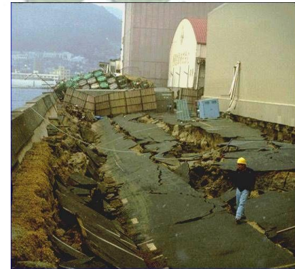
Fig. 9 Kobe earthquake - Japan (1995) Source: https://goo.gl/Xhgtif
