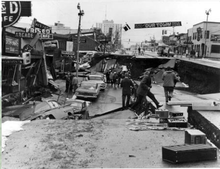
Fig. 8 Earthquake of Alaska - USA (1964). Source: https://goo.gl/uNTxW1
