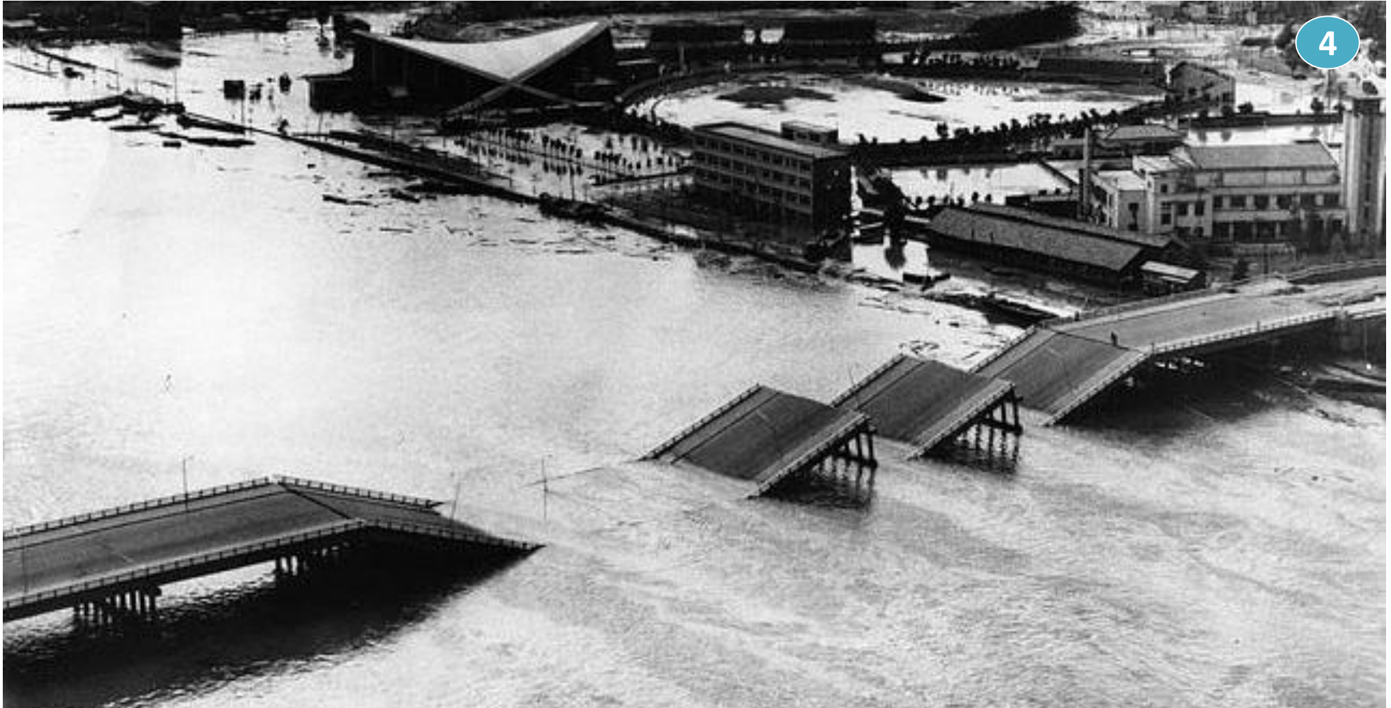
Fig. 6 Failure of Showa bridge boards. Source: https://goo.gl/LLvR5t
